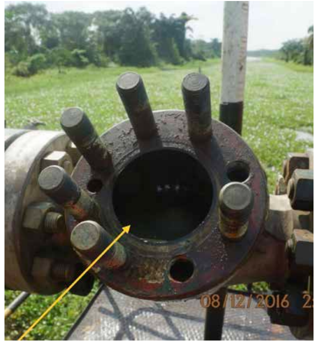
Close up of Shell's Benisede Well 6S Wellhead at Ojobo, where the company said unknown persons had stolen a "surface safety valve" causing a spill on 30 November 2016. Shell photograph.
