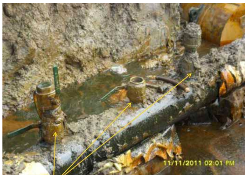
← Oil theft points on Shell's 12" Imo River - Ogale pipeline on 13 November 2011. Shell photograph.
