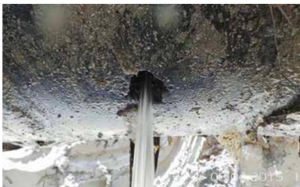
Leak point at Eni's 24" Ogoda/Brass pipeline (2015) . Eni photograph.
