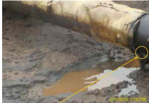
Leak point at the Ubie Well 9s Flowline at Idu/Edrass (2012). Shell photograph.
