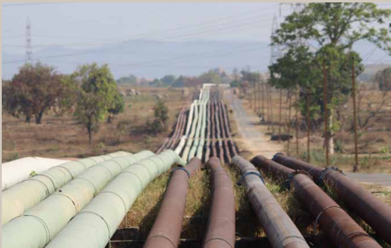
Pipes carrying slurry mixed with fly ash from Korba's thermal power plants criss-cross the landscape. The plants draw coal from SECL's mines, April 2014. © Amnesty International India
