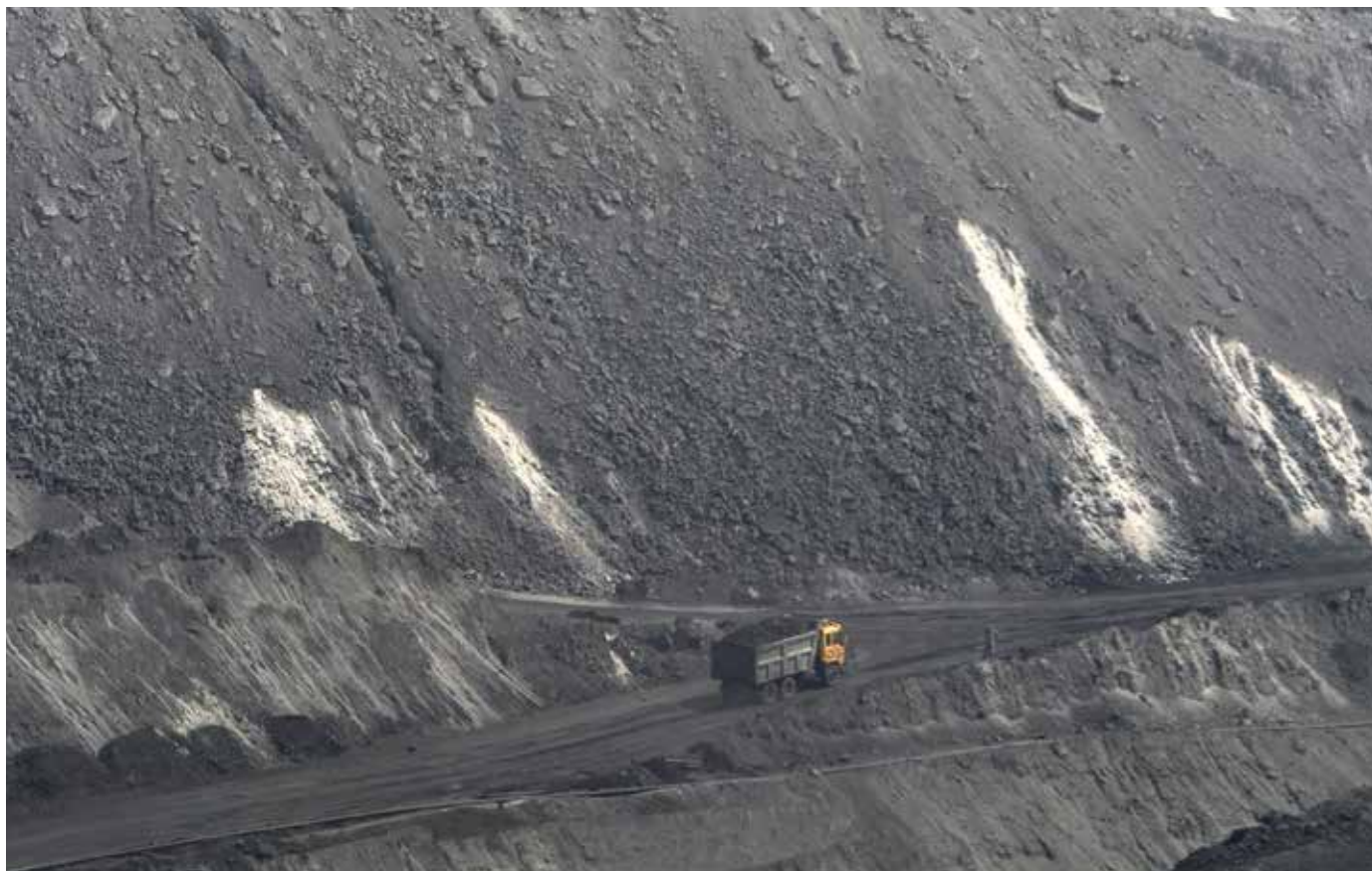
Kusmunda Open Cast Mining Project, Korba, Chhattisgarh, as seen from Barpali village, April 2014. © Amnesty International India
