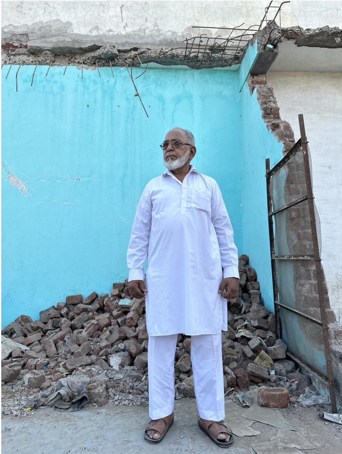
Khargone, Madhya Pradesh: Rafiq Shaikh stands in front of his demolished shop.
