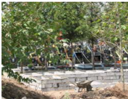
New individual burial plots being constructed over the suspected site of mass graves in Tazeh Abad cemetery. © Akhbar Rooz
