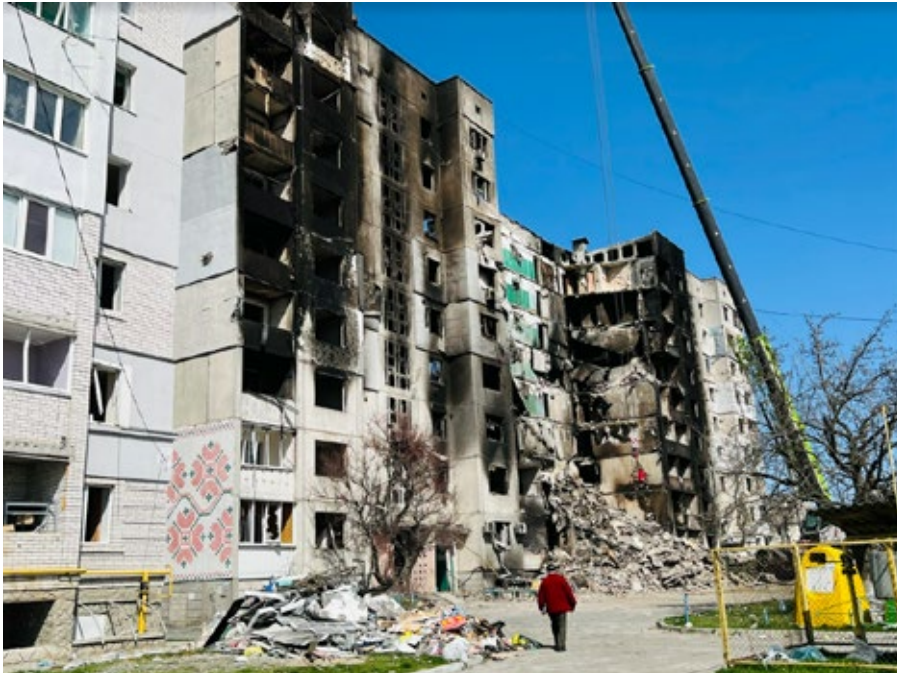
👁️ ← Building 353, which was bombed on 2nd March 2022 in Borodyanka. © Amnesty International
